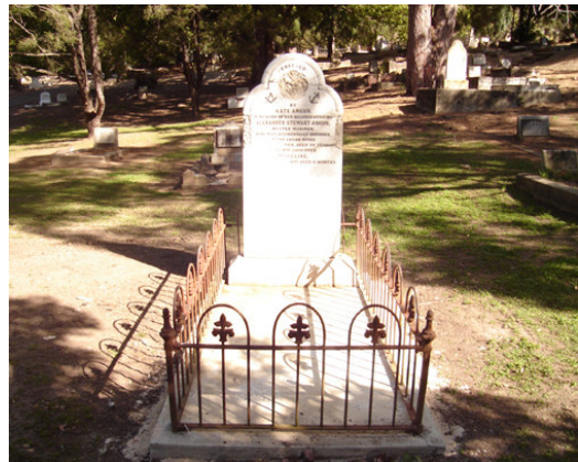
After restoration work had been completed
